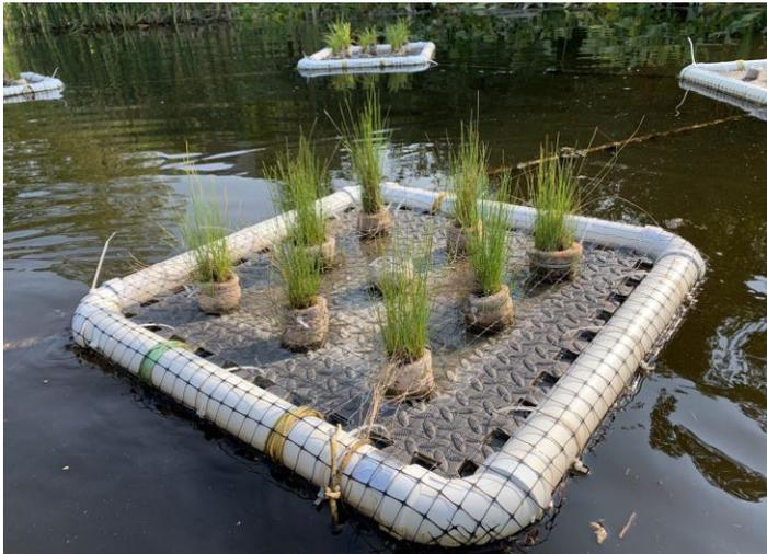
*Figure 2.16.* Design of constructed floating wetland adopted from Chen, Z. & Costa, O. (2020).
