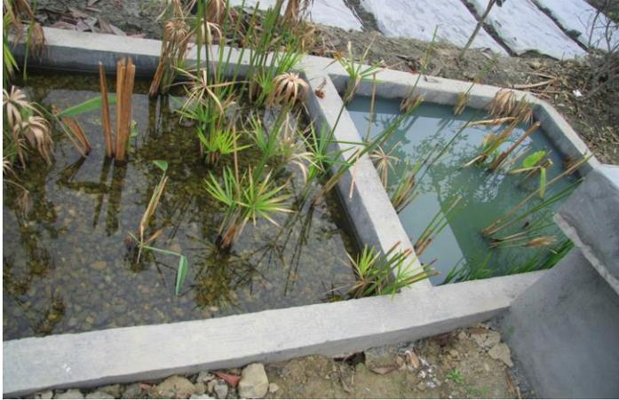
*Figure 2.15.* A constructed wetland made with concrete blocks. Photo by WWF-China/Chen Chan.
