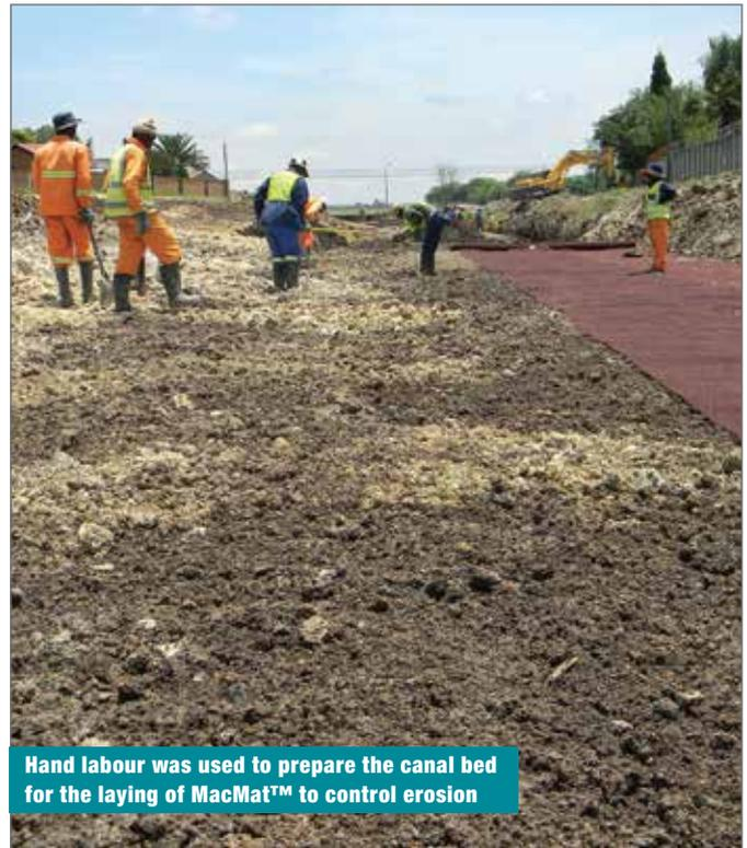
Hand labour was used to prepare the canal bed for the laying of MacMat™ to control erosion
